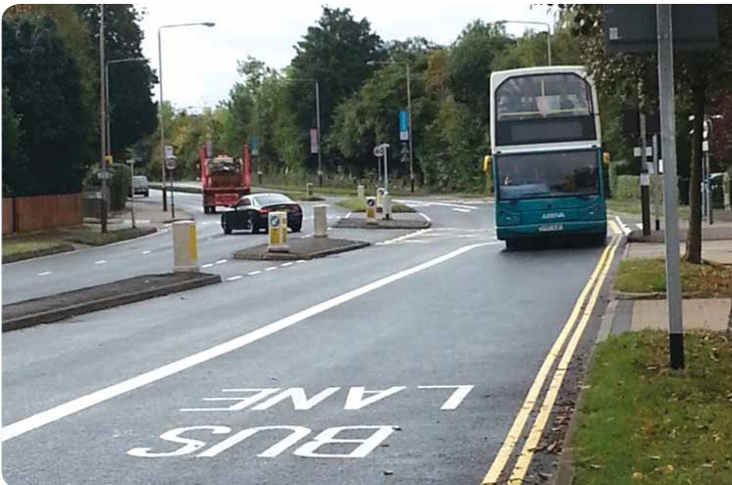
A426 Aylestone Road corridor
